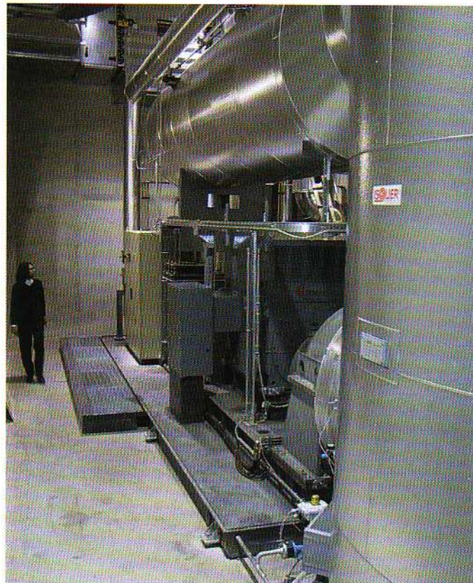
Turboden 1100 kW ORC cogeneration unit commissioned in March 2002 at Bregenz, Austria
