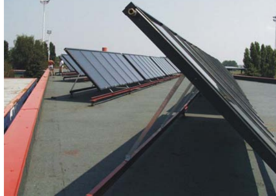
Collectors on the roof during the installation phase
