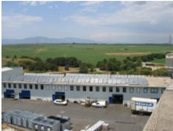
View of collectors filed in MEVGAL plant
